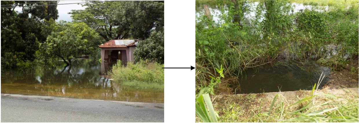
Figure 5.13: Flood Waters from the Pond and Neighbouring Flooded Properties Leading stormwater across the road via small culverts
