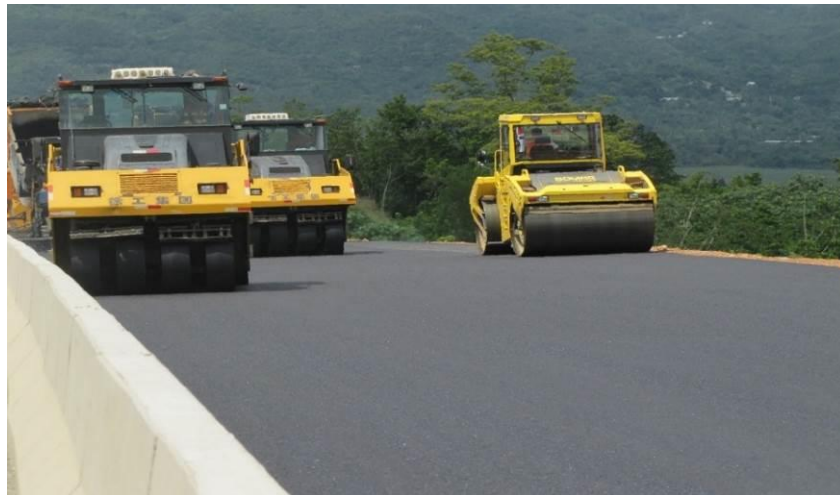
Figure 1.14: Spreading of Asphalt Concrete
