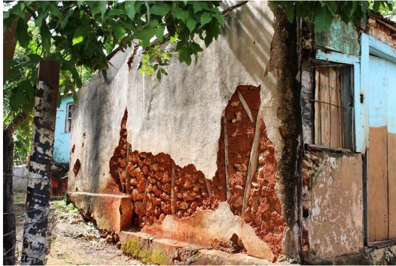
Figure 4.90: Wattle and Daub Structure in Upper St. Toolis
