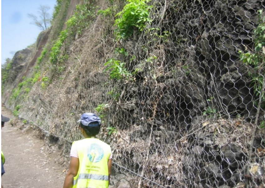
Figure 5.1: Example of Net Mesh Construction for Rock Fall Protection
