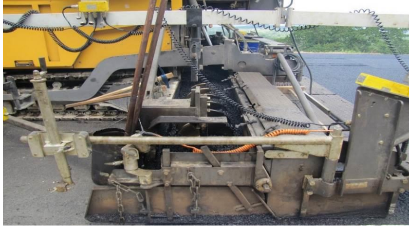
Figure 1.13: Spreading and Compacting Asphalt Concrete
