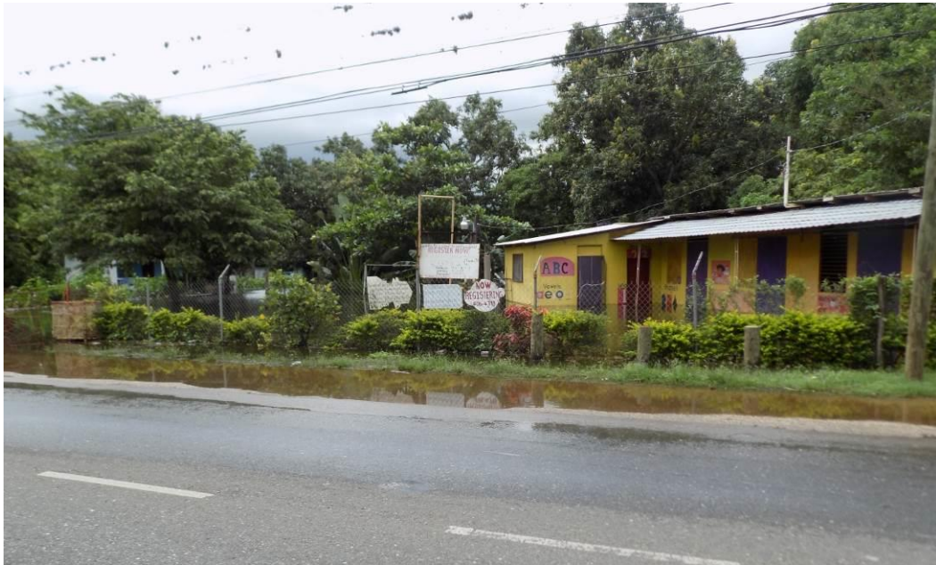
Figure 5.14: Flooding of school grounds adjacent exiting road
