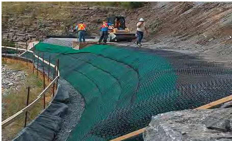
Plate 9.10 - Geogrids being placed on face of slope
