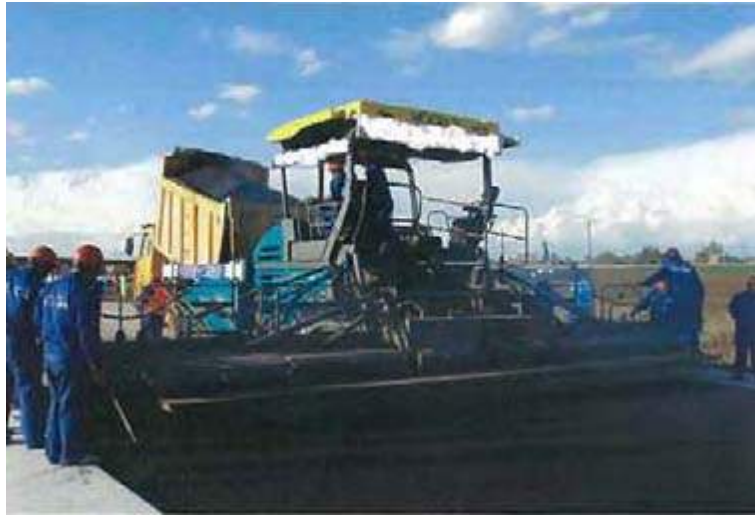
Plate 2.3 -Asphalt Concrete Spreading (source CHEC)
