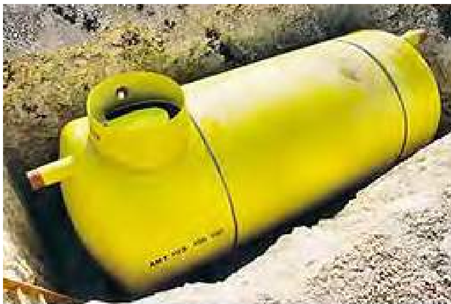
Plate 9.2 - Filling station forecourt separator
