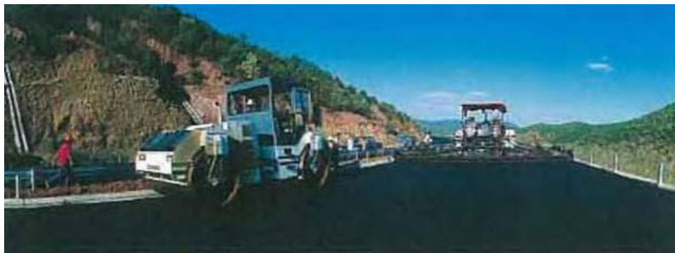
Plate 2.4 - Spreading and Compacting Asphalt Mixture (source CHEC)
