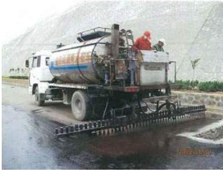
Plate 2.1 - Asphalt Pavement Construction (Spraying) (source CHEC)
