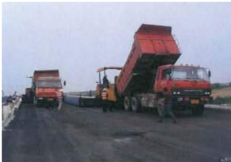
Plate 2.2 - Transportation of Asphalt Concrete (source CHEC)
