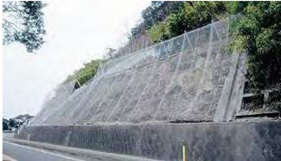
Plate 9.1 - Rockfall catchment fences being implemented
